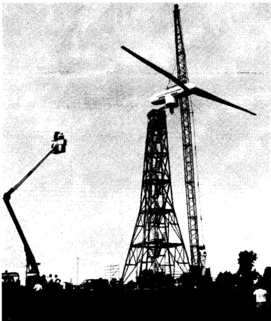
Under construction in the fall of 1975, the original Mod-O wind turbine had a rigid truss tower with a central stairway (soon removed because it blocked the wind), aerospace blades and a 100-kilowatt rating.
