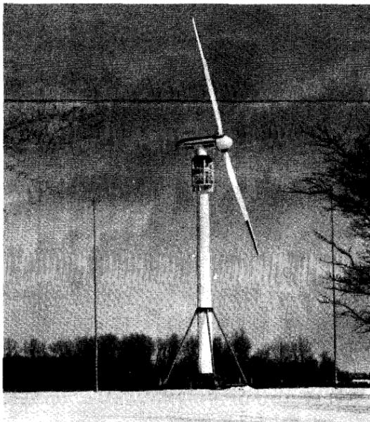
Research led to major changes to reduce weight, cost and complexity. By 1982 the tower was a flexible, low-cost cylinder; blades were made from laminated wood; and aileron control surfaces eliminated the need to pitch the entire blade to control power and speed.
