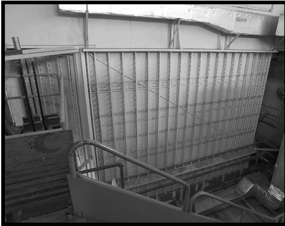
Figure 34.—Wall built between the high bay and the test chamber for the Near-Field Antenna Test Facility, 2007 (OH_Cuyahoga_AWT-Support_034).
