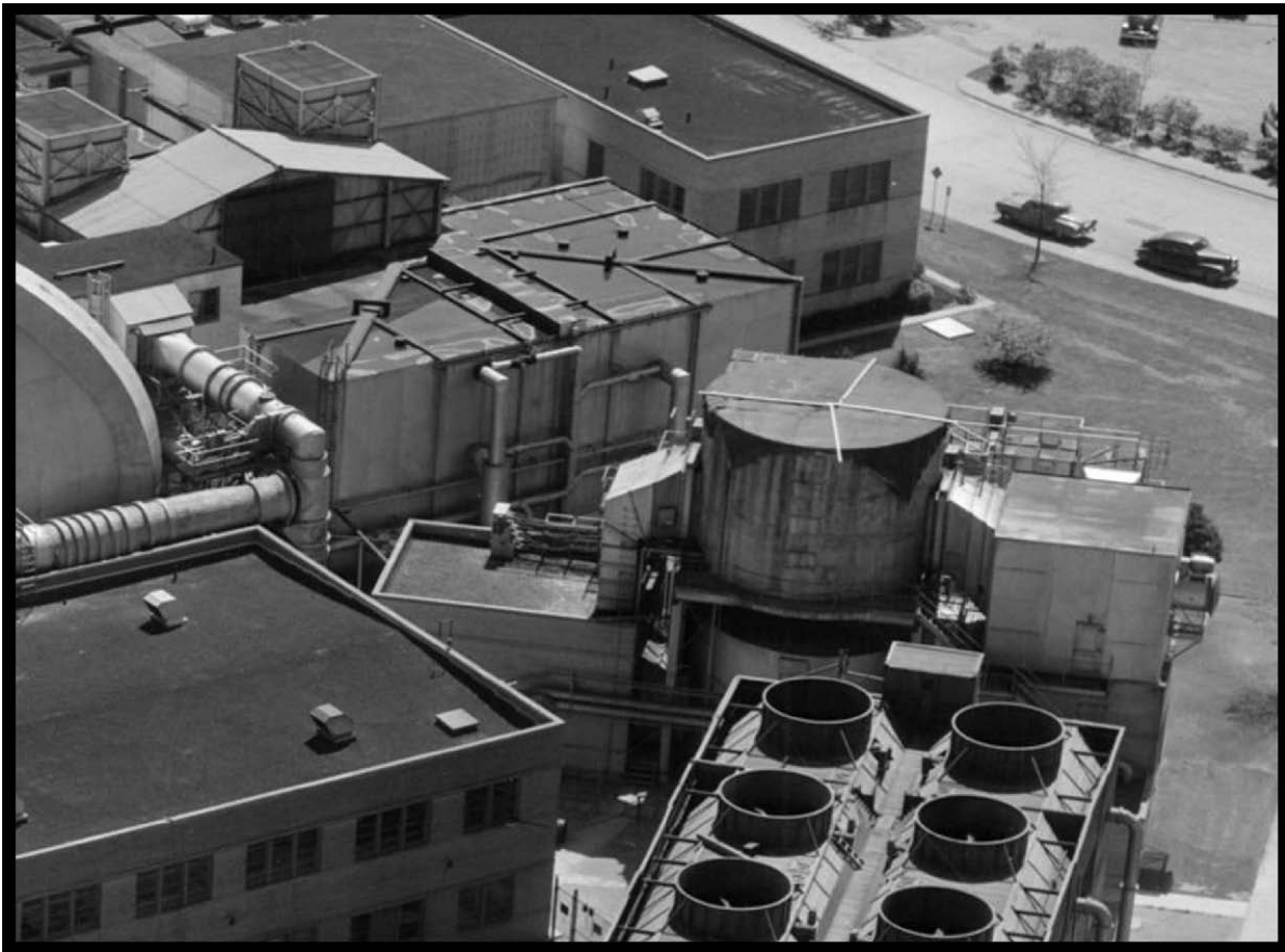
Figure 78.—Air Dryer Building after a new dryer tank and primary coils were added on top (viewed from the northwest), 1955 (OH_Cuyahoga_AWT-Support_078).
