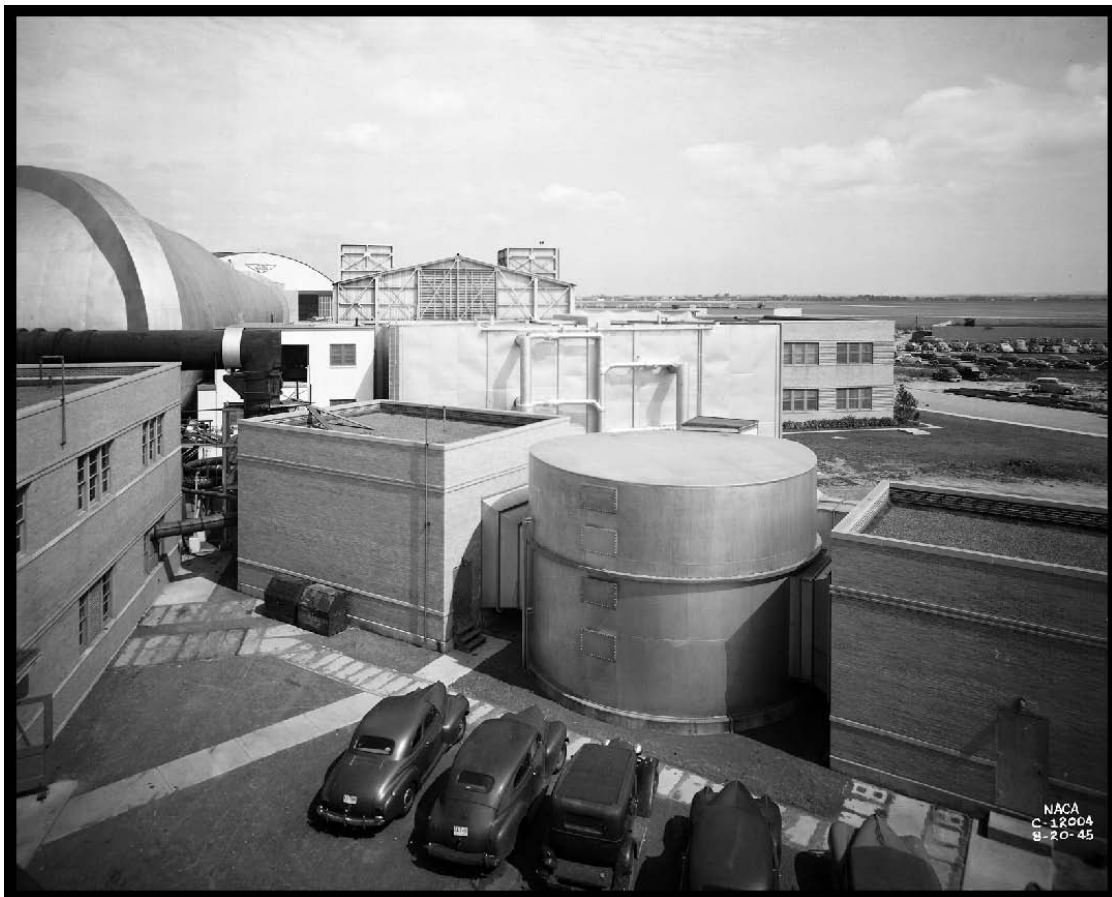
Figure 77.—Original air dryer setup with the secondary coils (left), dryer tank (center), and primary coils (right) (viewed from the west), 1945 (OH_Cuyahoga_AWT-Support_077).
