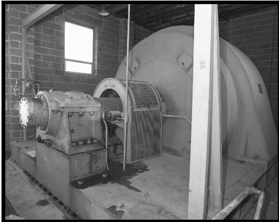
Figure 52.—General Electric induction motor that was used to drive the AWT fan (viewed from the northeast), 2005 (OH_Cuyahoga_AWT-Support_052).
