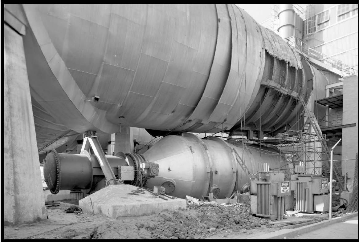
Figure 68.—Installation of the exhaust gas cooler under the northeast tunnel section during the upgrade of the AWT, 1951 (OH_Cuyahoga_AWT-Support_068).
