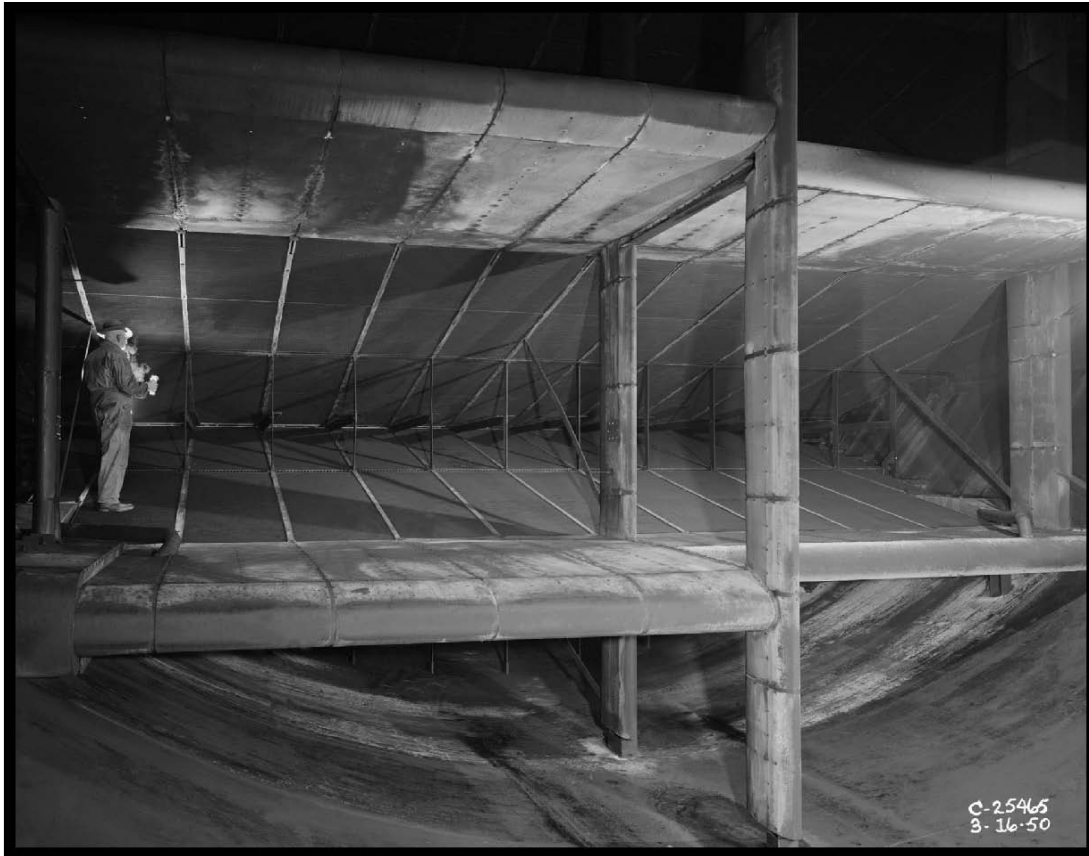
Figure 62.—Accordion-shaped banks of cooling coils inside the AWT, 1950 (OH_Cuyahoga_AWT-Support_062).
