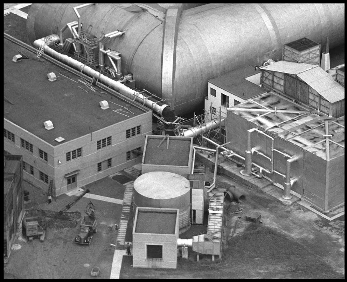
Figure 81.—Air Dryer Building showing air pipes feeding the AWT (left) and the Small Supersonic Tunnels (right) (viewed from the southwest), 1945 (OH_Cuyahoga_AWT-Support_081).
