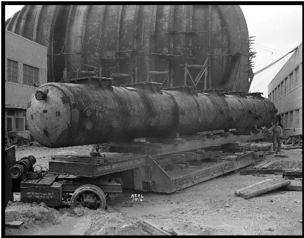
Figure 60.—Flash cooler being prepared for installation in the Refrigeration Building in July 1943 (OH_Cuyahoga_AWT-Support_060).
