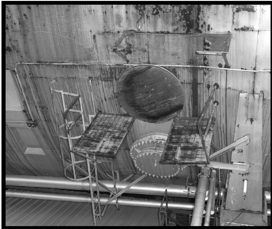
Figure 86.—Portals in the south leg of the AWT where the Small Supersonic Wind Tunnels formerly tied in, 2005 (OH_Cuyahoga_AWT-Support_086).
