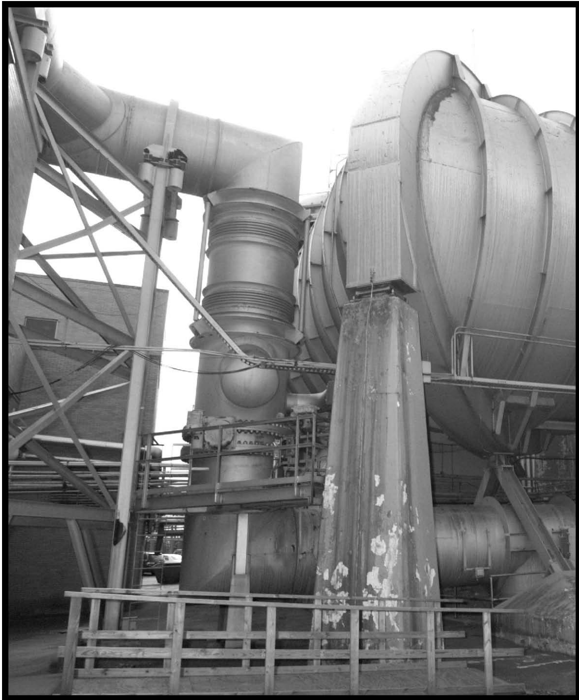
Figure 69.—72"-diameter pipe connecting the cooler pit to the Exhauster Building and the ERB, 2005 (OH_Cuyahoga_AWT-Support_069).
