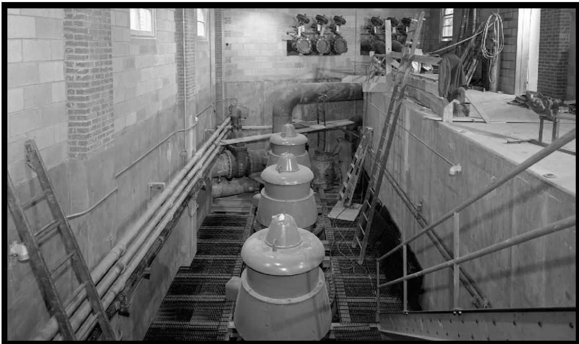
Figure 67.—Three of four sump pumps inside the Circulating Water Pump House during its construction in 1951 (OH_Cuyahoga_AWT-Support_067).
