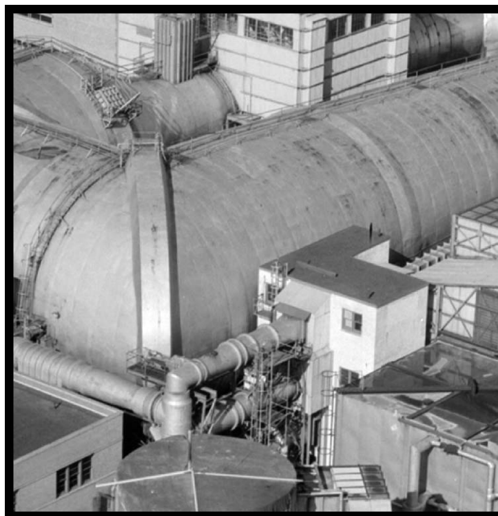
Figure 83.—Line from the air dryer feeding the Small Supersonic Wind Tunnels (viewed from the southwest), 1955 (OH_Cuyahoga_AWT-Support_083).
