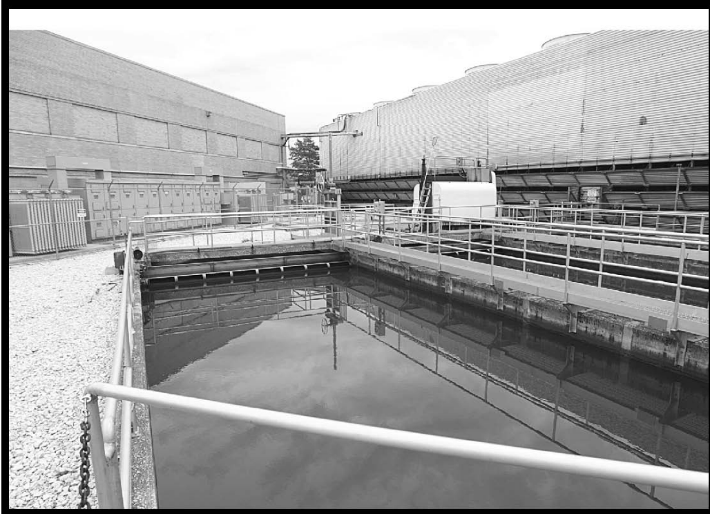
Figure 76.—Cooling Tower No. 1 with its settling basins in the foreground (viewed from the northwest), 2005 (OH_Cuyahoga_AWT-Support_076).
