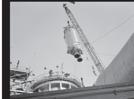
A Centaur 6A rocket is lowered into the Space Power Chambers' vacuum tank for a series of environmental tests. The Centaur's auxiliary propulsion, hydraulic, pneumatic, and electrical systems were tested during long periods in a space environment. The chamber could simulate an altitude of about 100 miles, and create the cryogenic temperatures and radiant light of space.
