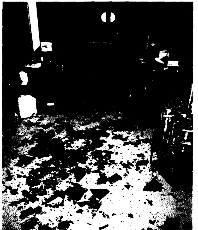
ABOVE: In 1985, an implosion in a cooler in the basement of the Engine Research Building was caused by the failure of several welds between a support beam and the cooler floorplate. RIGHT: The force of the implosion shattered windows and caused other damage to the building. The system's collapse may have been prevented if the insufficient welds had been identified and corrected earlier.
