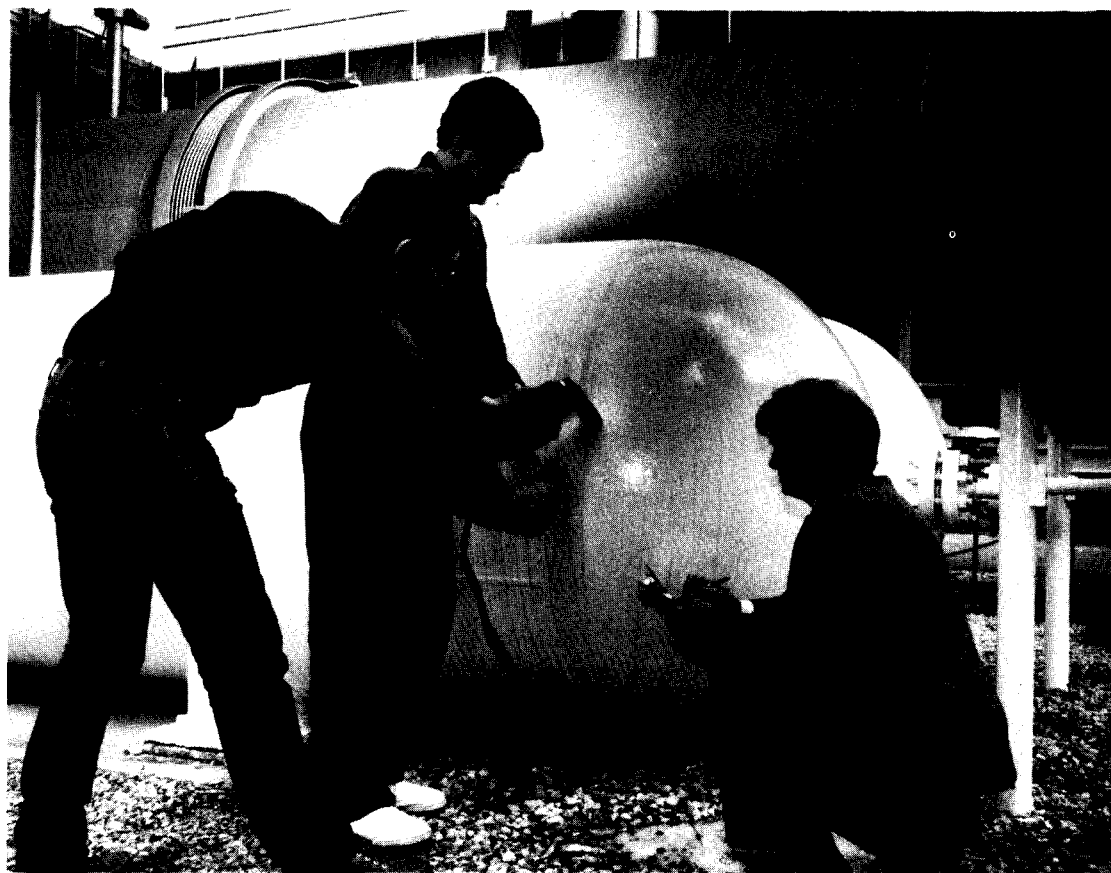
The current five-year recertification program is designed to insure the structural integrity and evaluate the remaining life of each of Lewis' 117 pressurized systems, 416 pressure vessels, 27 altitude exhaust coolers, 638 relief devices, and 360 expansion joints. Shown above: Recertification Program Manager Jim DeRaimo (kneeling) and O'Donnell and Associates employees Lou Hass (left) and Gary Selier conduct a magnetic particle inspection of a head-to-shell weld on a pressure vessel.
