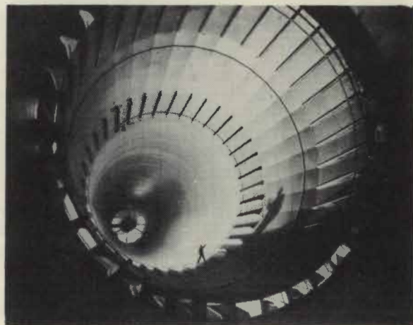
Cooling vents of 16-foot transonic tunnel
