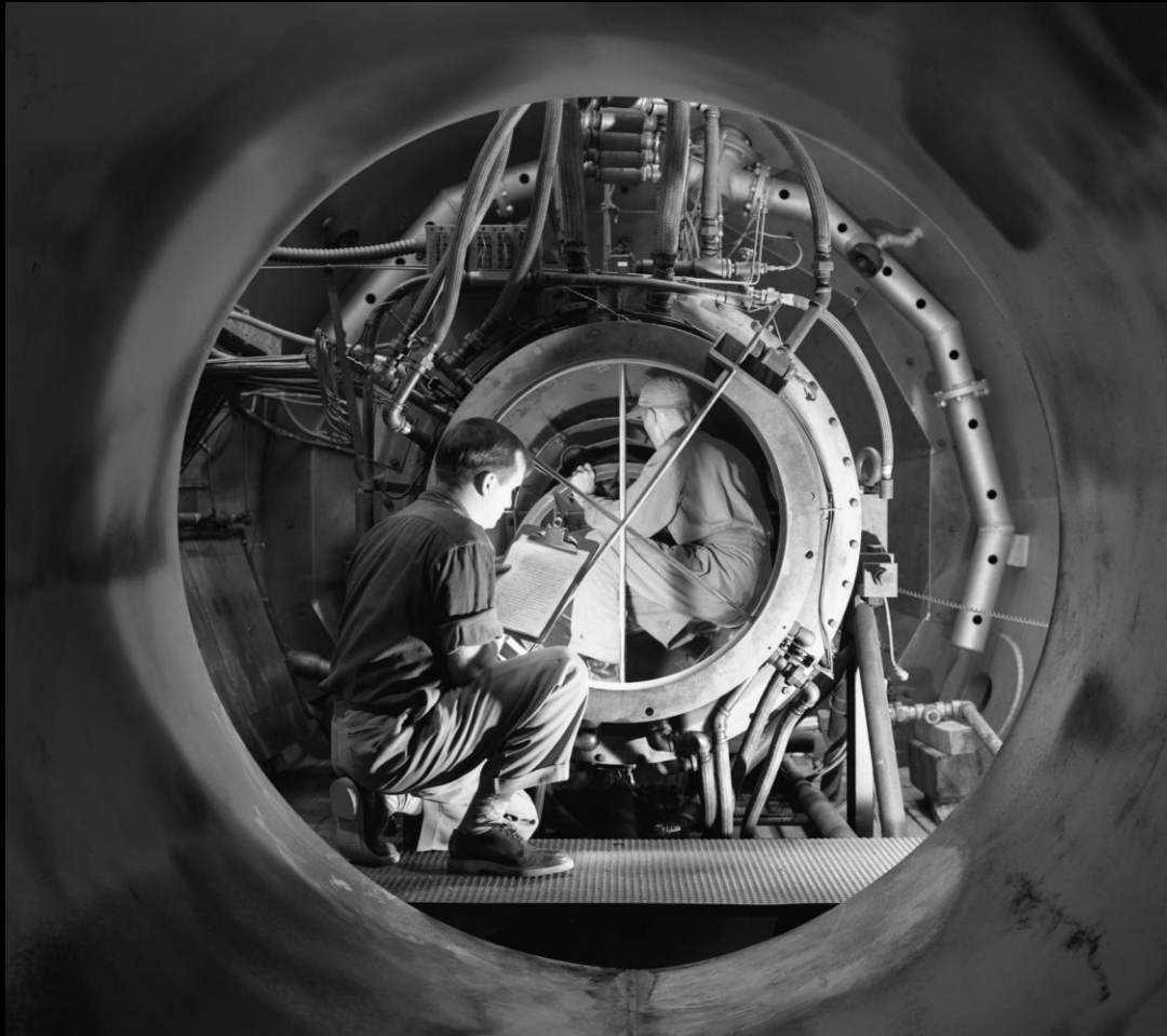
Technicians install a 48-inch ramjet in PSL No.1
