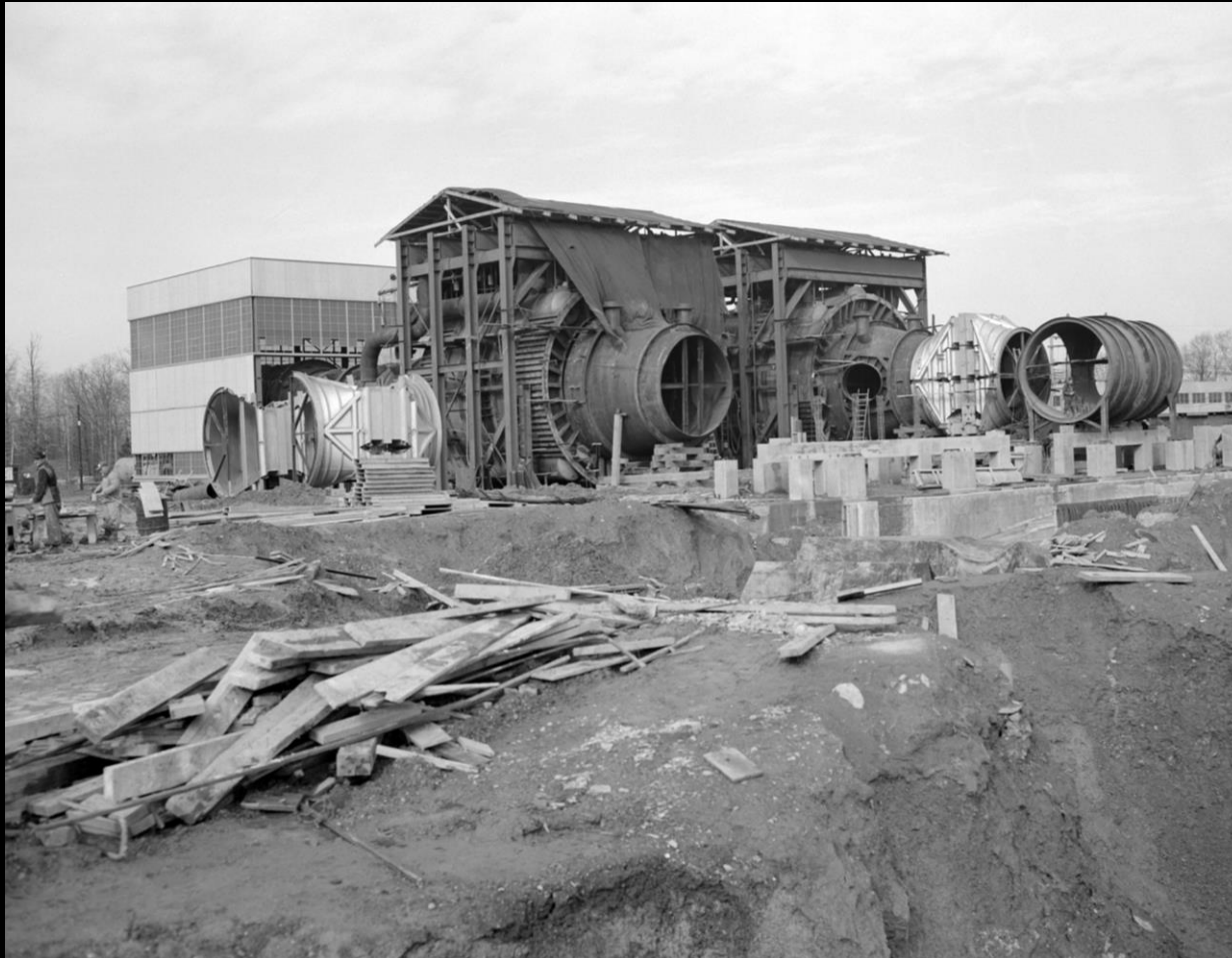
Construction of PSL No. 1 and 2
