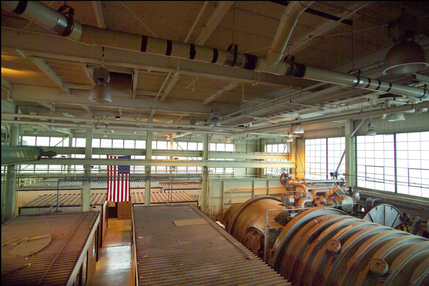
PSL No. 1 and 2 interior today
