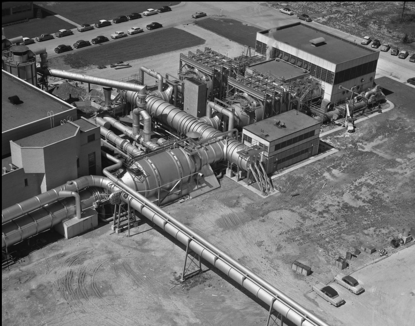
Propulsion Systems Lab No. 1 and 2
