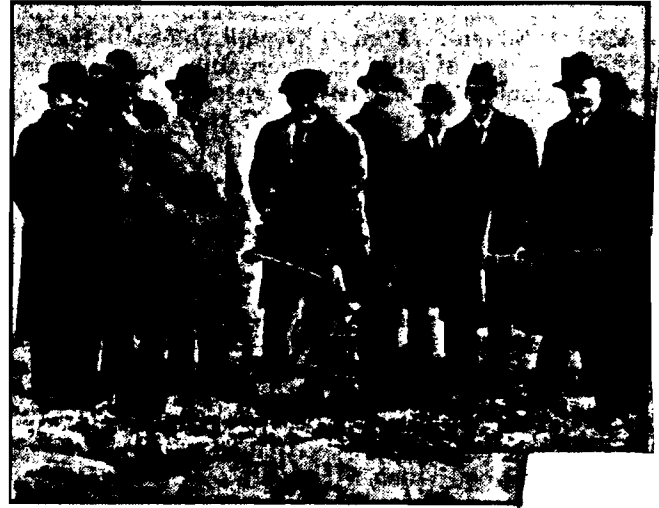
Above: A photograph of the January 23, 1941 groundbreaking ceremony at the then NACA Aircraft Engine Research Laboratory. Edward R. Sharp is third from the left. (Photo credit: NASA) Right: The pick and shovel from the groundbreaking ceremony now on display at the Edward R. Sharp Employee Building at the Glenn Research Center. (West Life photo by Kevin Kelley)
