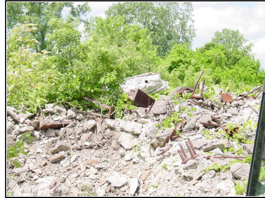
PHOTO 2 (Construction Debris Pile Rubble at FR-5)
