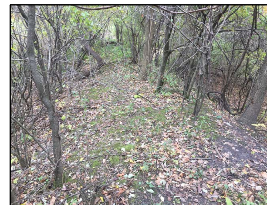
PHOTO 7 (Top of FR-5 Impact Berm)
