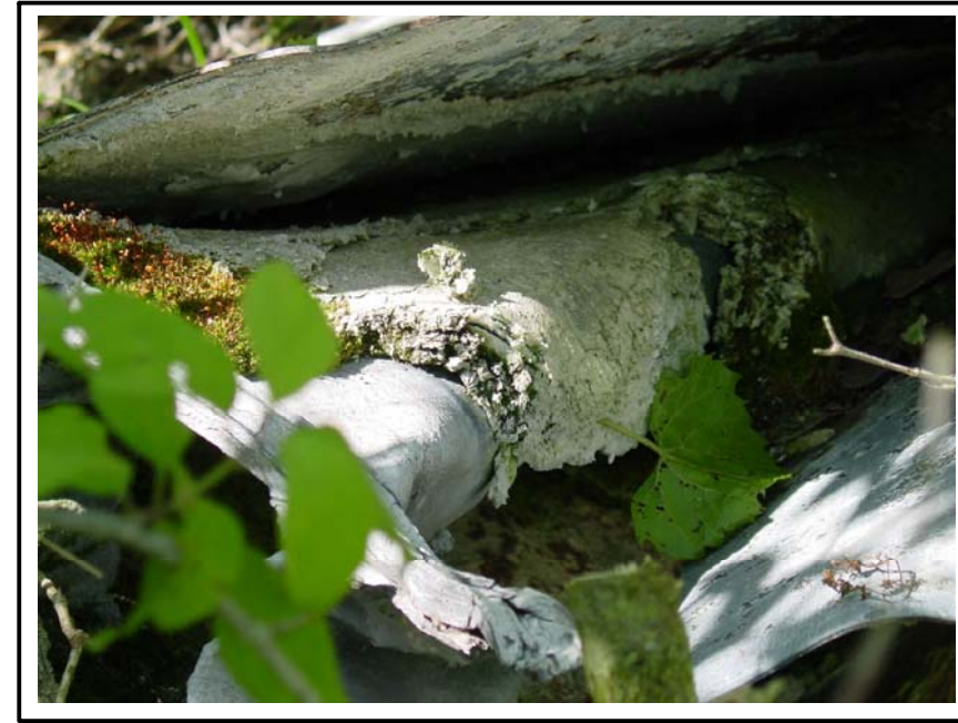
PHOTO 3 (Lead-Covered Asbestos Panels found in Construction Debris Pile)
