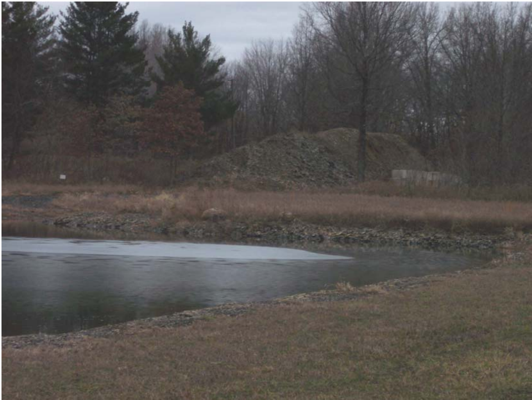
Photo 5. Shallow Pond Looking Southwest, Back of Impact Berm
