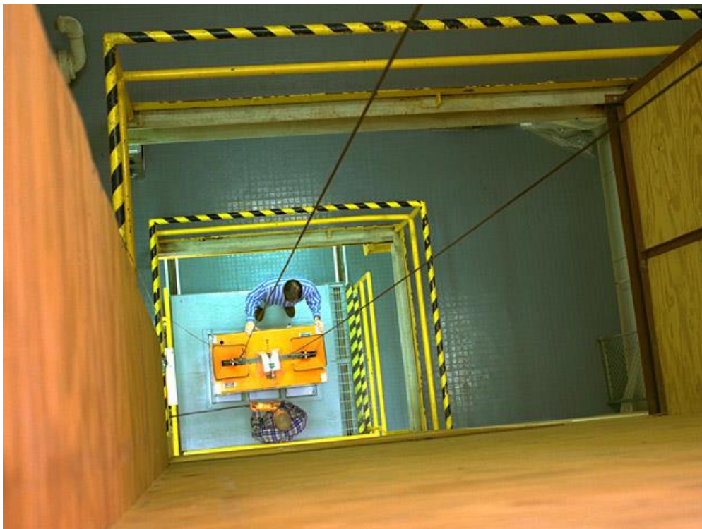
View from the eighth floor as technicians ready the drag shield assembly.
