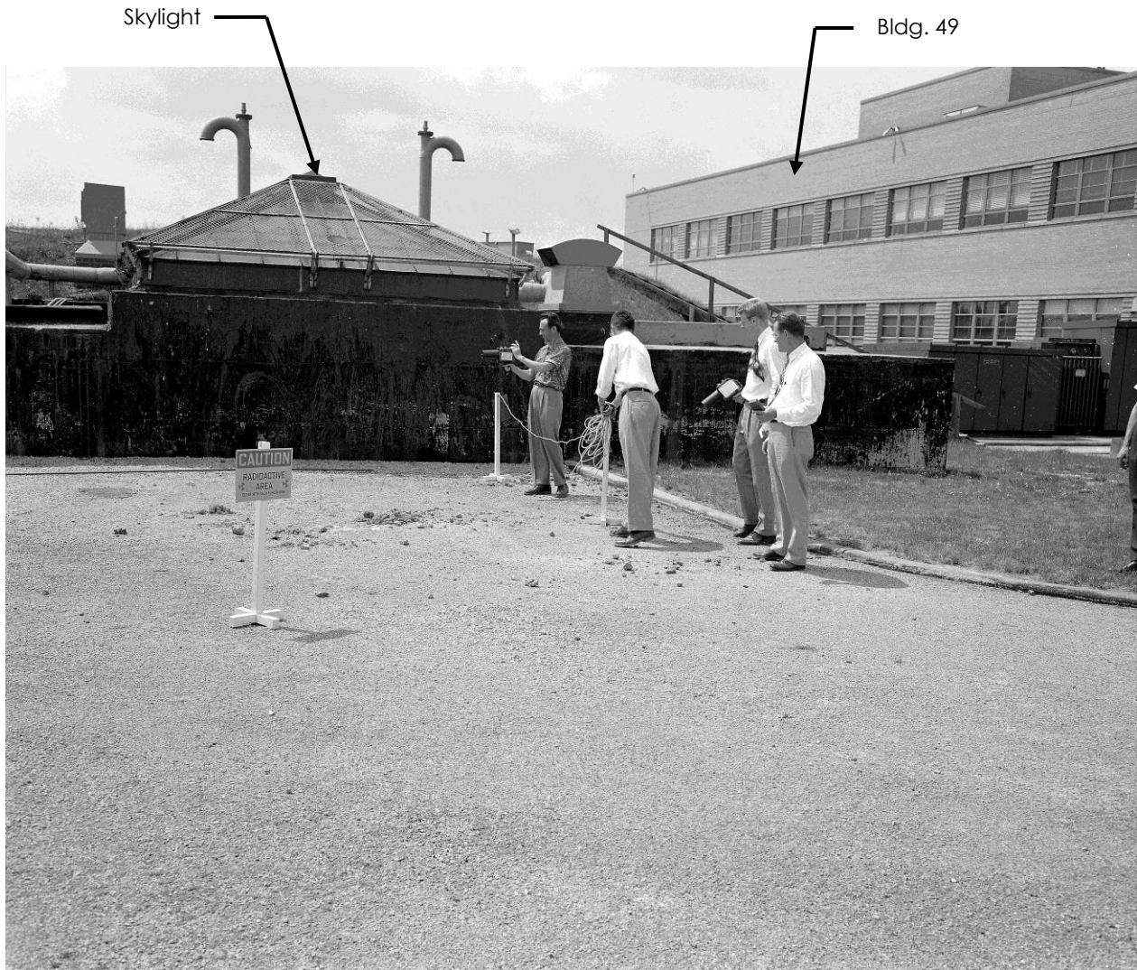
HISTORIC PHOTO East View over Sump Pump Pit, Work Area and Hot Storage Room
