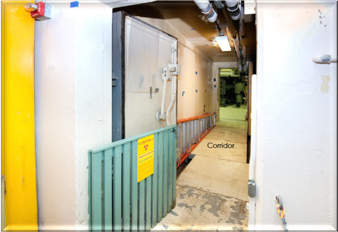
Entry into Cyclotron Facility from Bldg. 49 Basement
