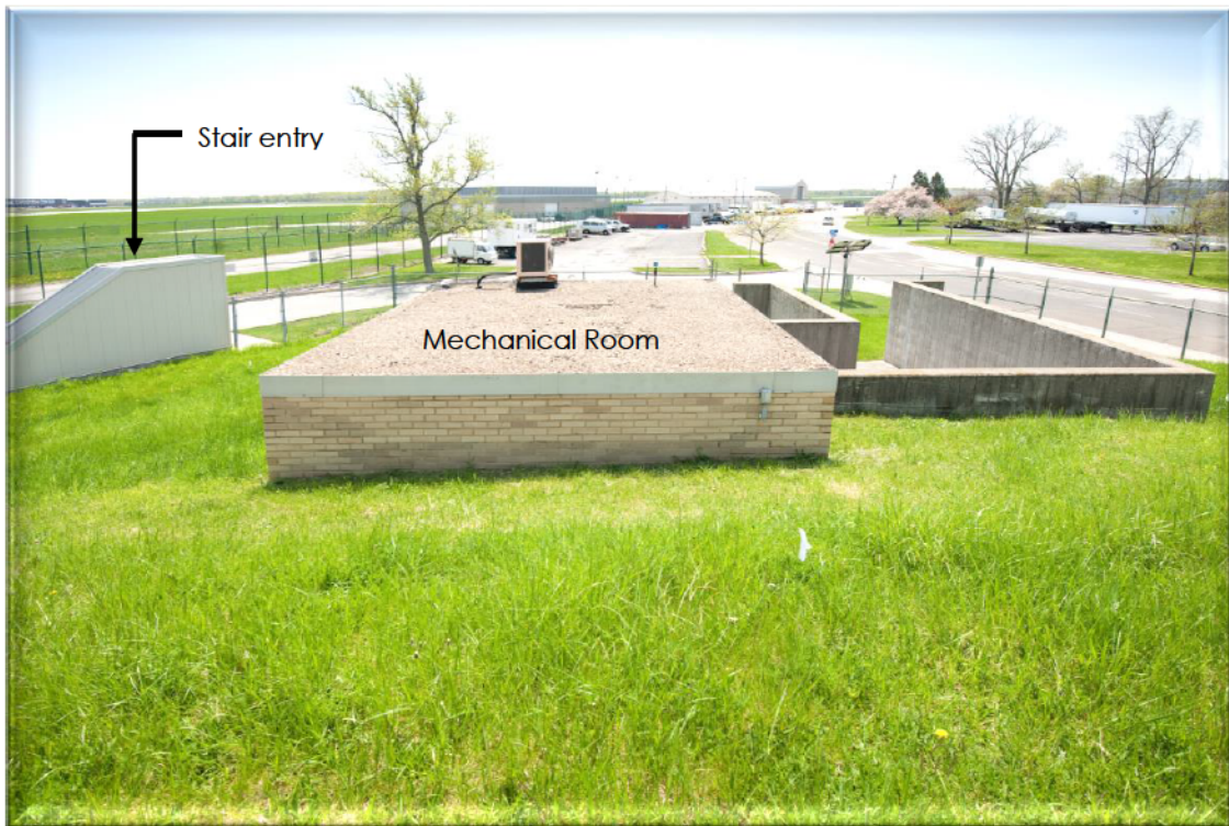
Roof top view of Mechanical Room and retaining walls around drive Photo 2
