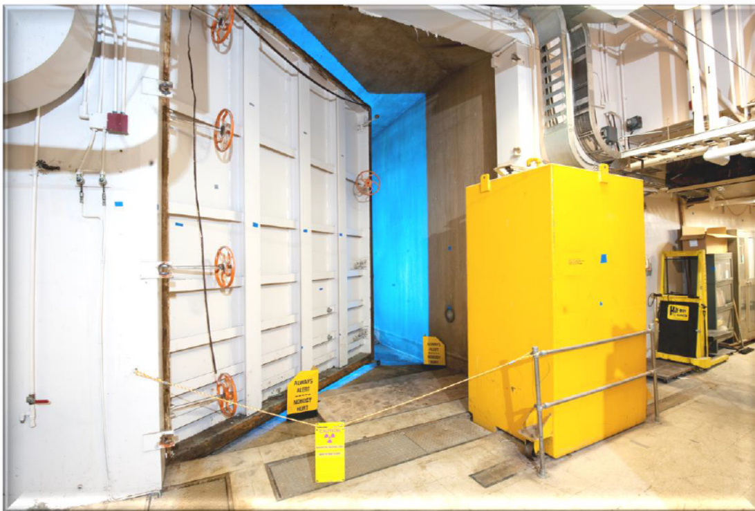
Door into the Vault Room where the Cyclotron is located
