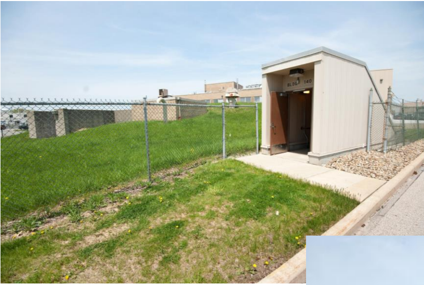
Stair entry into Cyclotron below Photo 5
