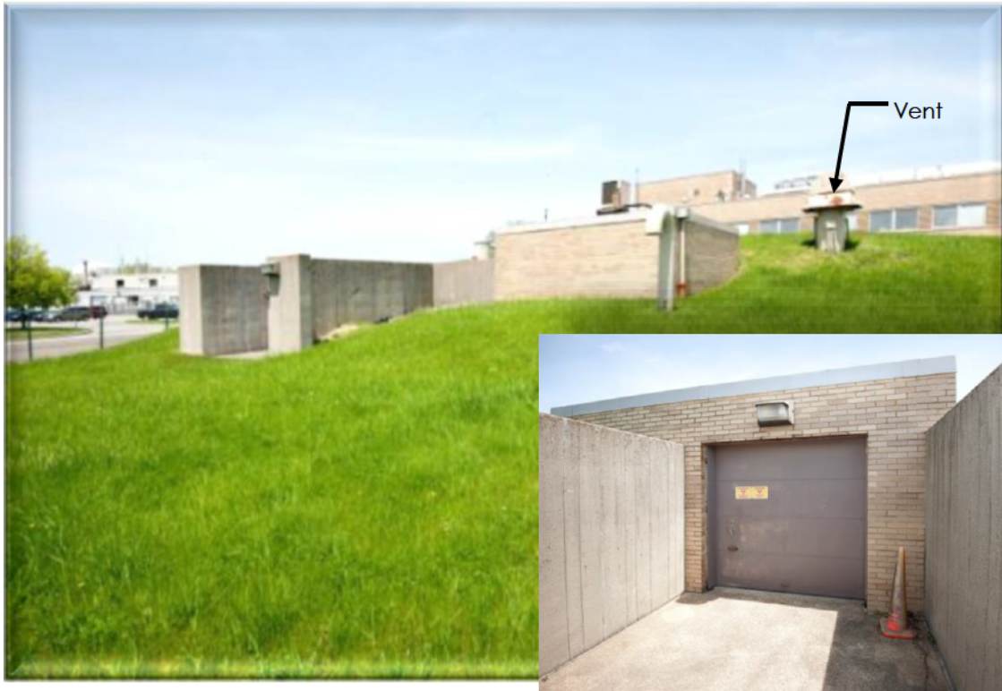
View of above ground Mechanical Room overhead sectional door Photo 3
