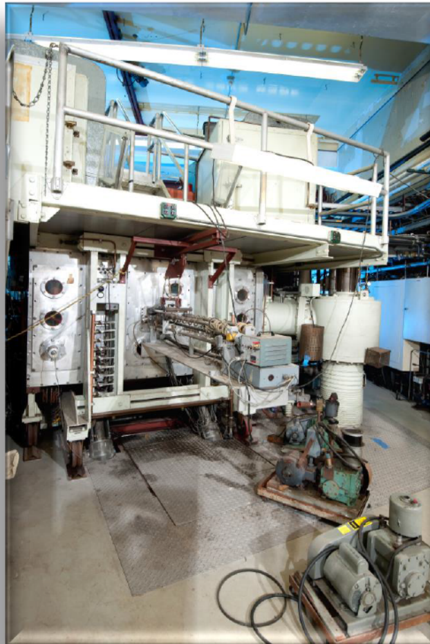
Rear View of Cyclotron
