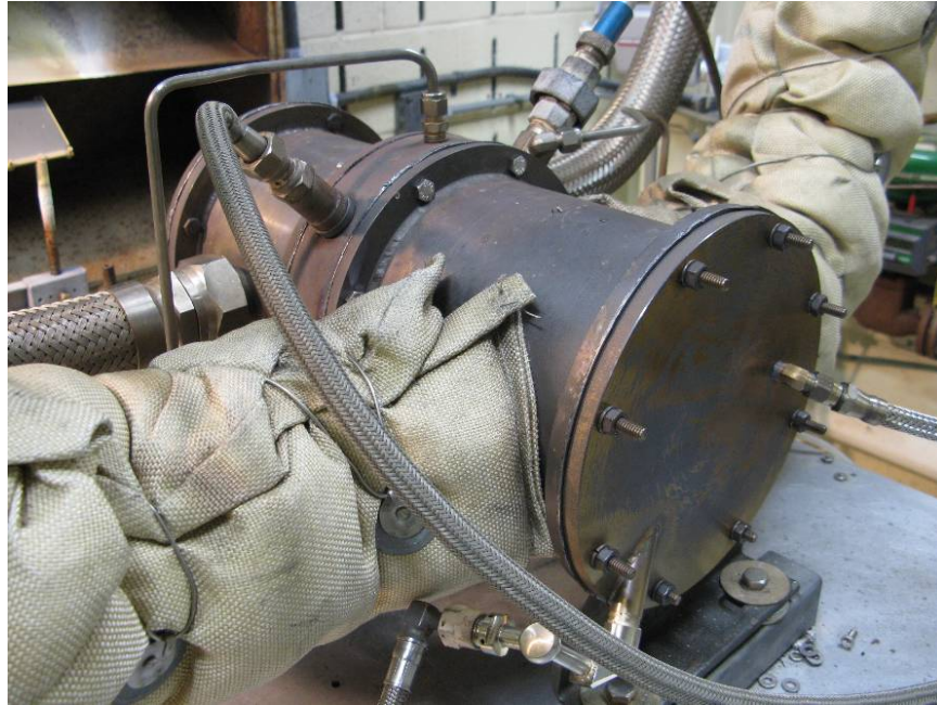
Figure 17.—Fuel nozzle plate installed. Braided hose in plate leads to a pressure tap.
