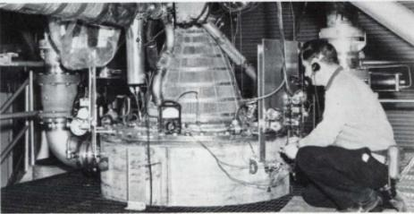
**COMPLETED EXPERIMENTS** — Tests with flight-weight NERVA-type nuclear reactor engines and a rocketed engine regeneratively cooled, nozzles were conducted at the B-3 facility. Radioactive fuel elements were not used in the engine during tests. Here, an electrician checks wiring connections for one of the many remotely operated valves prior to a test run. In space operation, this valve would feed liquid hydrogen to the reactor where it would be converted to gas and provide the rocket thrust.
