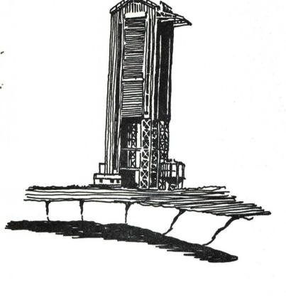
This \$3.5 million, 200-foot high, facility is used for non-nuclear altitude tests on various components for large nuclear rocket engines such as will be needed for interplanetary travel. A 46,000 gallon liquid hydrogen run tank is located in the tower, and liquid and high-pressure gas can be supplied by rail car. A 200,000 gallon liquid hydrogen supply tank is located in the front of this facility.
