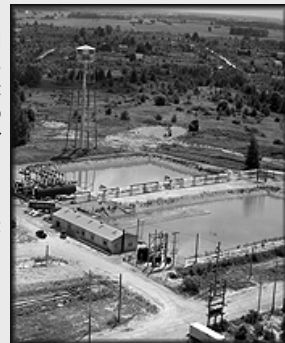
Pump and Shop Bldg
