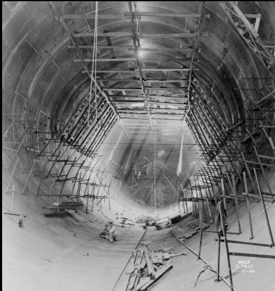
Interior of AWT during construction
