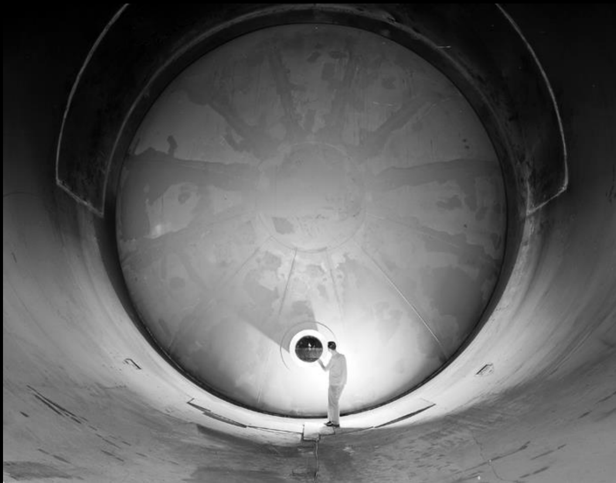
Bulkhead installed inside AWT
