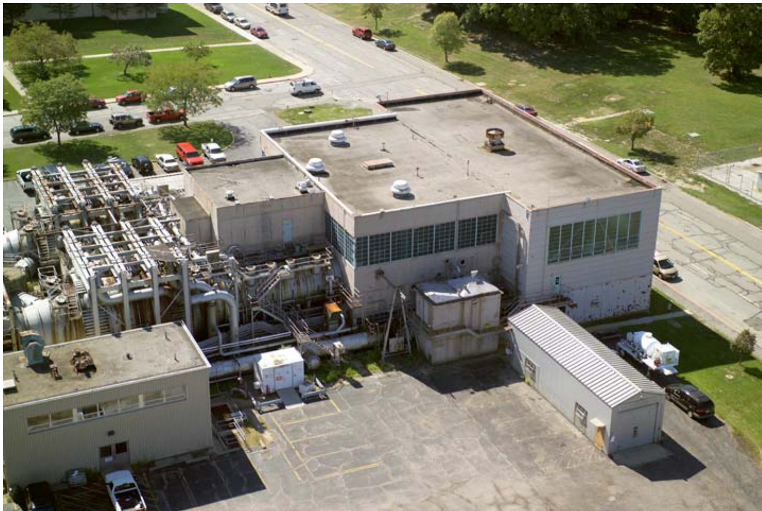
Photograph of PSL 1 & 2 Viewed from the North
