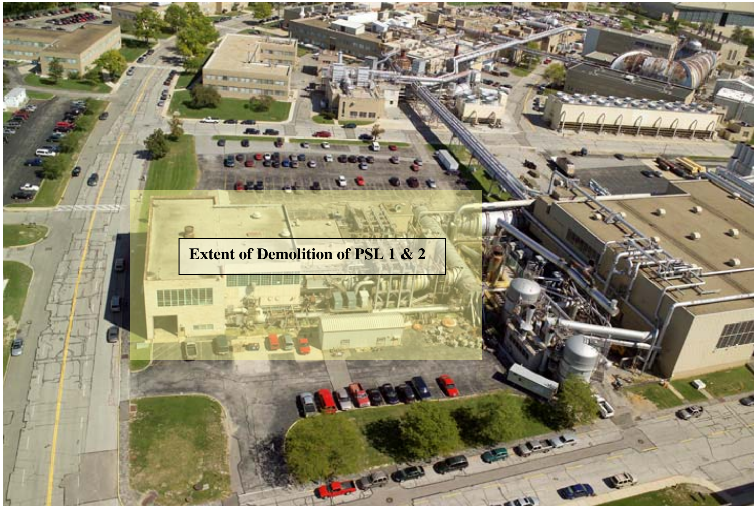
Photograph of PSL 1 & 2 Viewed from the South
